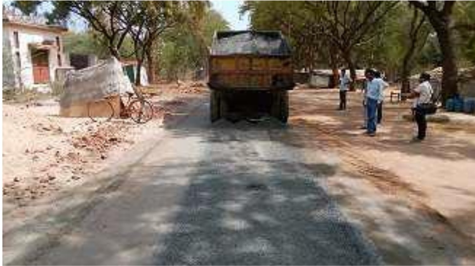
(Sample photograph-9 Grit spreading)
