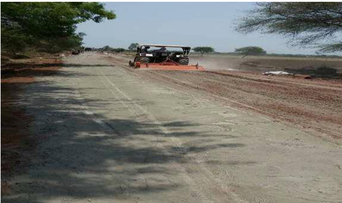
(Sample photograph-3 soil cement mixing with rotavator)
