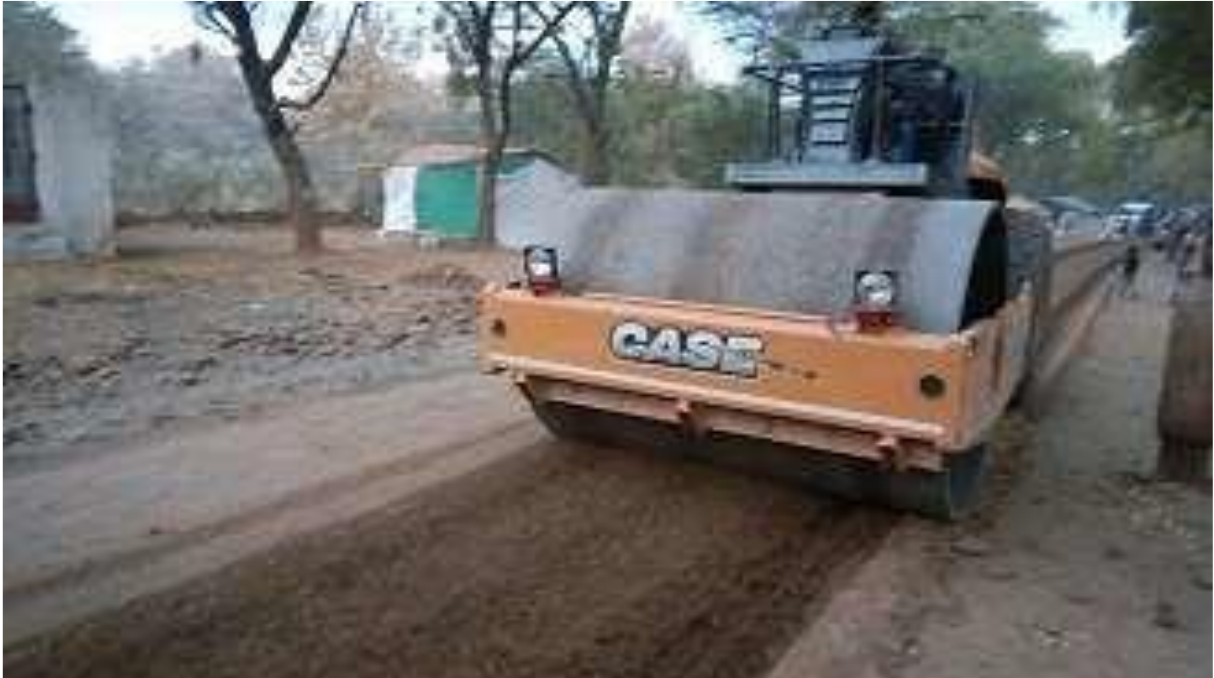
(Sample photograph-7 Compaction with Vibratory Roller)
