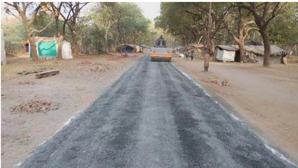
(Sample photograph-10 Compaction with Vibratory roller)
