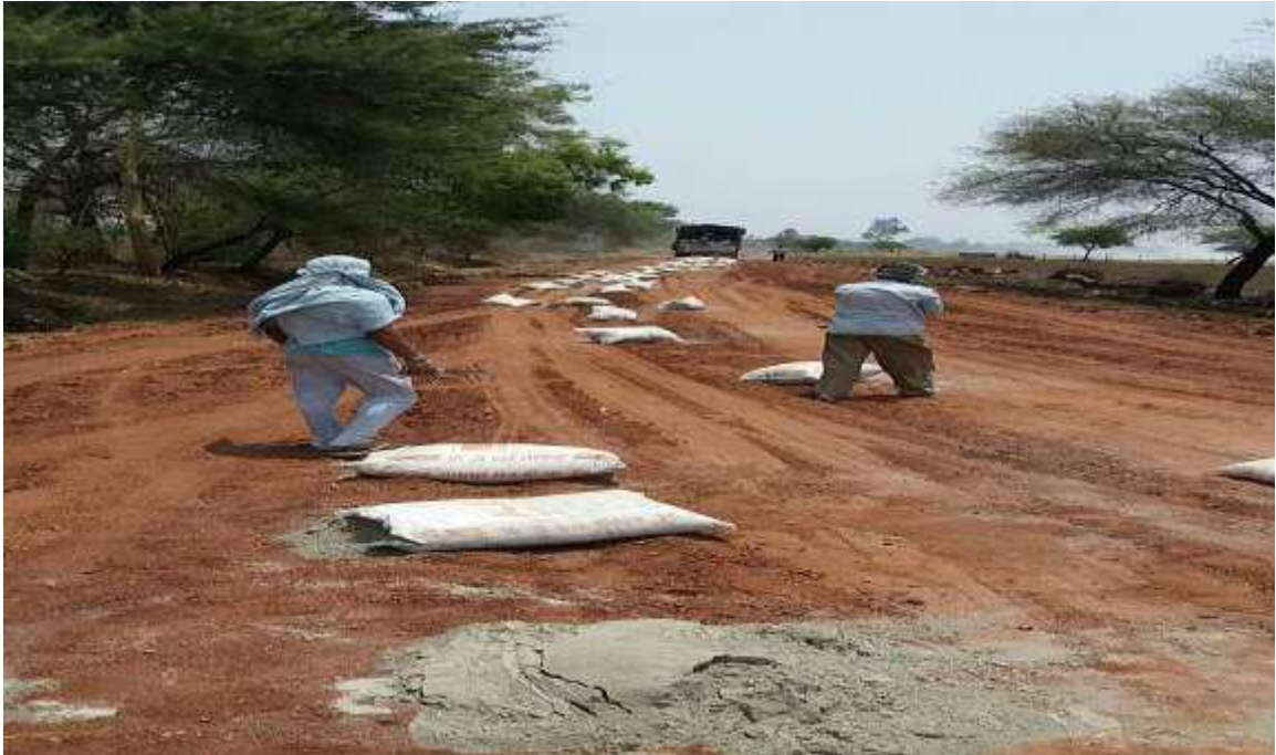
(Sample photograph-3 soil cement mixing with rotavator)
