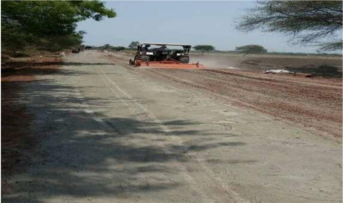
(Sample photograph-3 soil cement mixing with rotavator)
